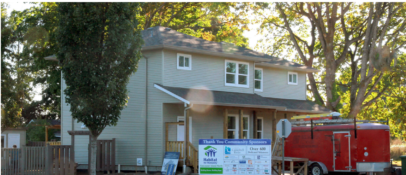
Our 2016 build project on Westgate Road in Campbell River.
