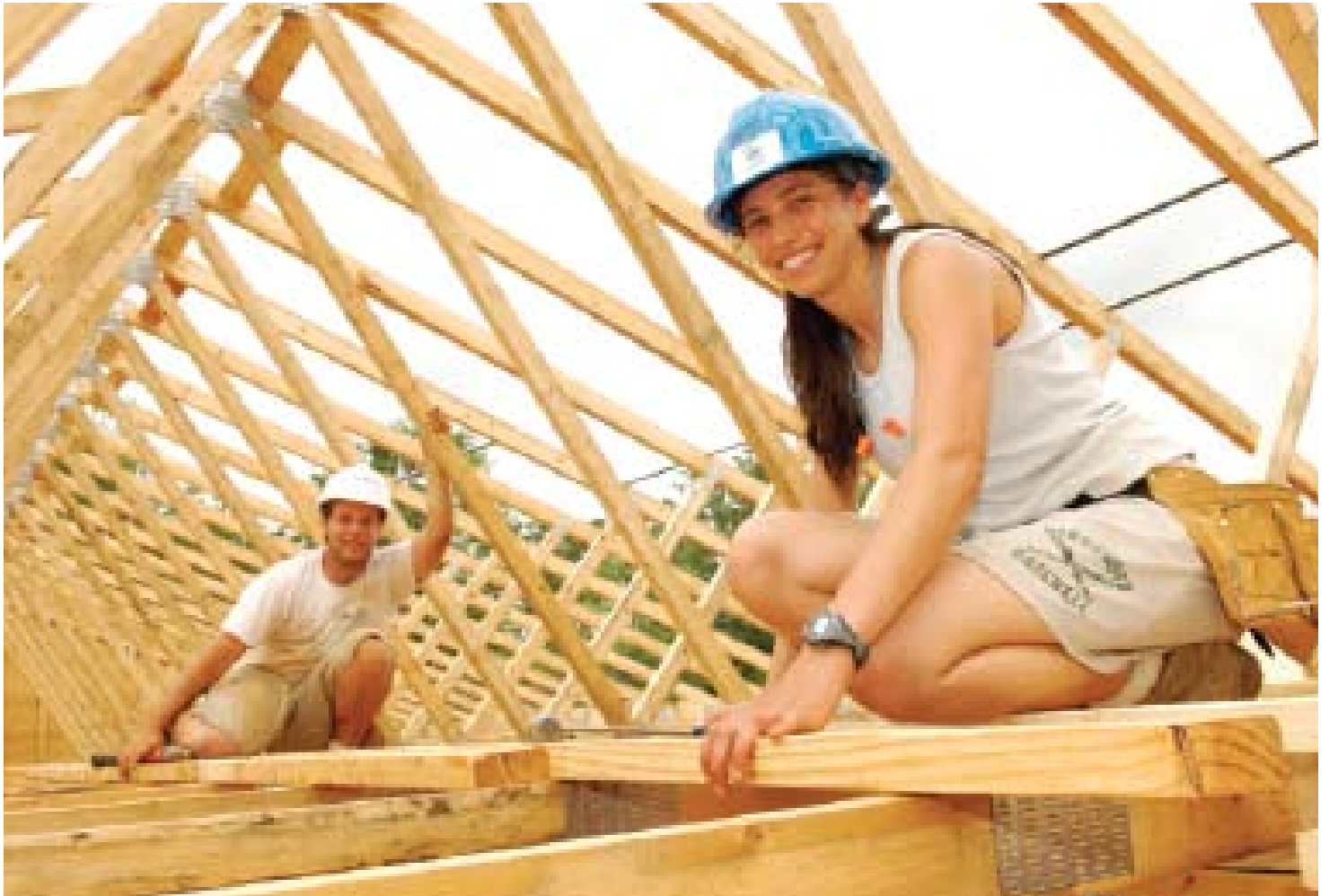
HABITAT VOLUNTEERS WORKING ON BUILDING A NEW ROOF.
